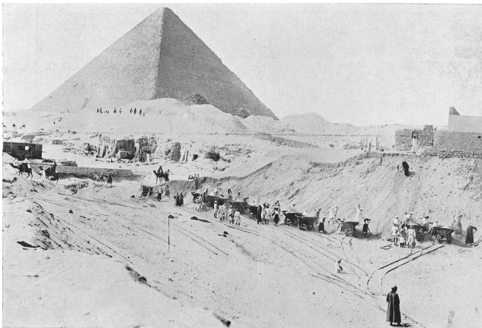
THE FIELD OF EXCAVATION LOOKING WEST. NOTE FAN-LIKE LAYING OF TRUCK RAILS
