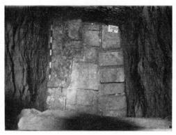
Masonry packing in shaft just before roof of chamber was reached; looking vertically down, March 7, 1925.
