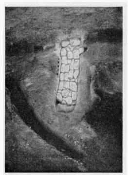
Masonry packing of stairway, after removal of plaster, February 20, 1925.
