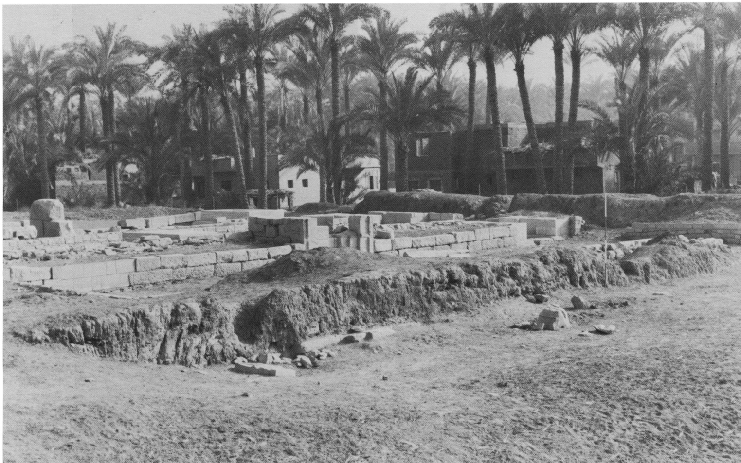
General view of the Apis House looking northeast. In the center is the niched recess in Wall CD; Table 4 is behind it, and the west jamb of Entrance AB is on the left.
