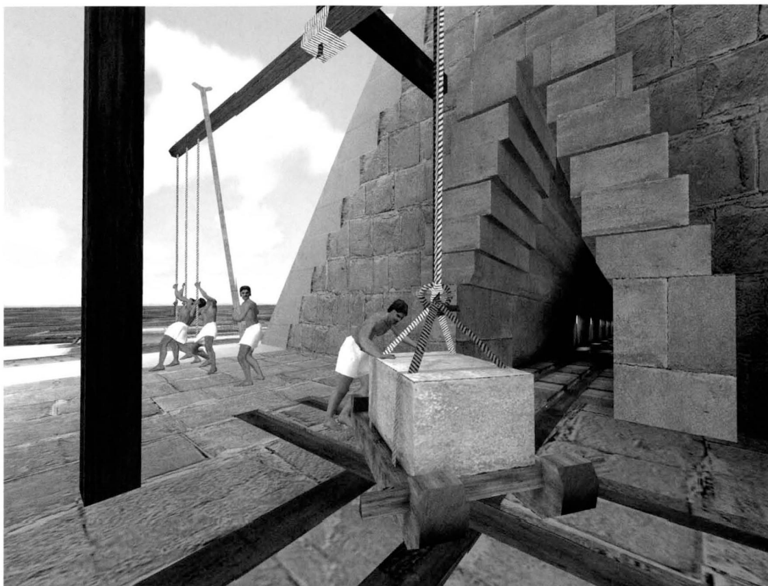
Fig. 4. Notches at the corners were left open to help turn the blocks with simple cranes. Photograph courtesy of Dassault Systèmes.
