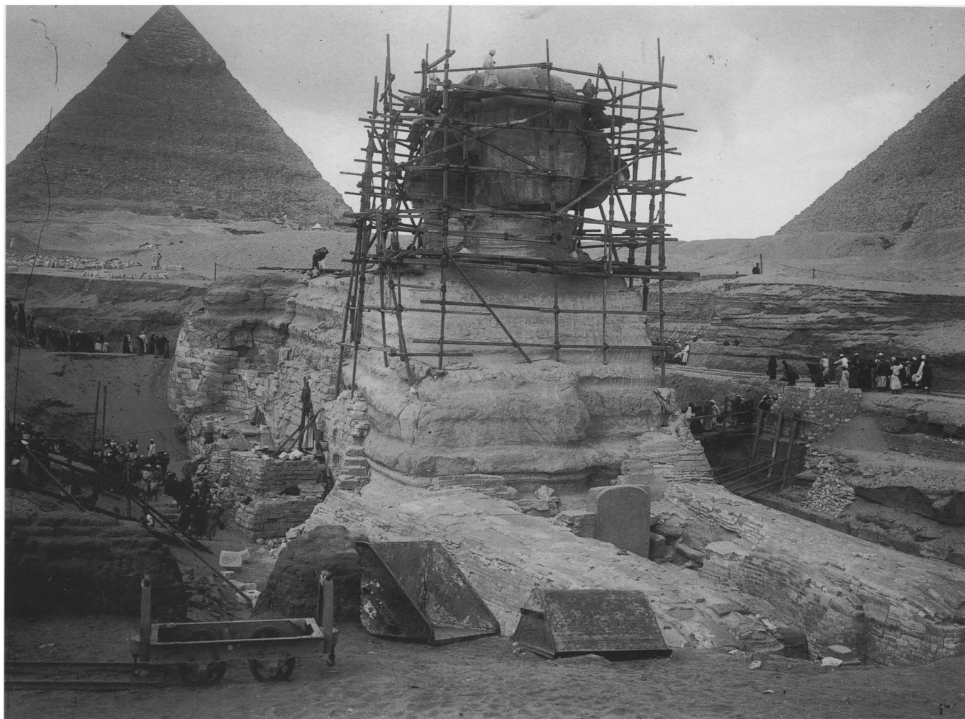
Fig. 90. The Great Sphinx, with the restoration scaffolding of Émile Baraize, looking northwest, December 26, 1925. The pyramids of Khufu (right) and Khafre (left) are in the background.
